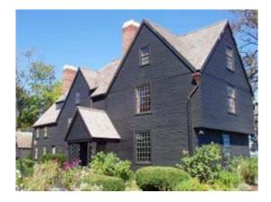
A **gable** is the triangular portion of a wall between the edges of a sloping roof. The shape of the gable and how it is detailed depends on the structural system being used (which is often related to climate and availability of materials) and aesthetic concerns. Thus the type of roof enclosing the volume dictates the shape of the gable.
